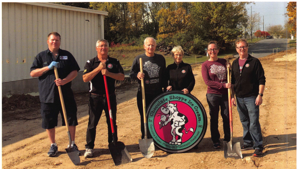
Groundbreaking for The Chocolate Shoppe Ice Cream's new ice cream mix plant. From left: Charlie Deadman, Chuck Deadman Jr., Chuck Deadman Sr., Nancy Deadman, Sarah Deadman, Dave Deadman.
